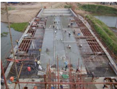
Concreting of the top part of box beam
