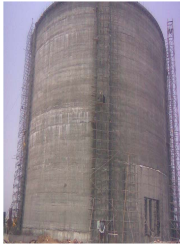
View of silo during final stage of stressing
