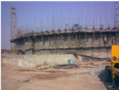
Silo view during slip forming construction
