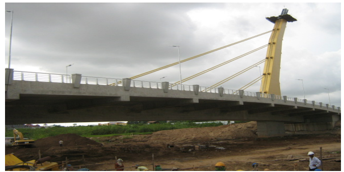
View of the Swan Bridge
