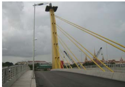
View of completed deck
