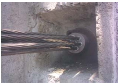
PBL anchorage M705 after stressing
