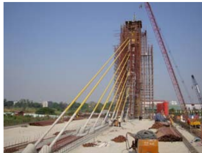
Cable duct installation
