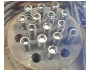
Spring over Cut Strand Protruding End Prior to Covering with Protection Cap at Dead end Anchorage Set
