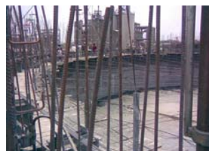
View of Silo Construction at Miryalguda
