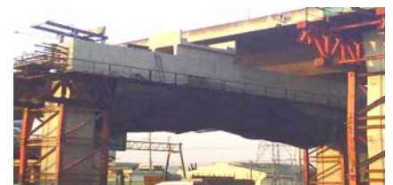
Beam on Left Side of Portion Frame after Concrete Casting
