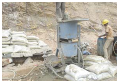
During grouting of Hill Rock Gaps
