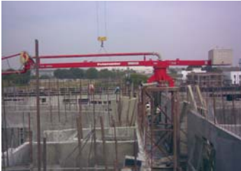
Rotary Concrete Placer for Slabs
