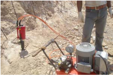
Pull Out Test of Mono strand anchor up to 140 KN
