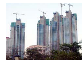
Millennium Residence under Construction
