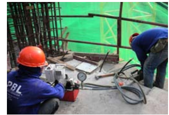
Stressing of PT Slab under Progress
