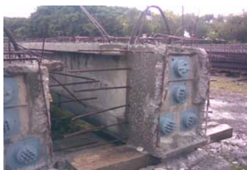
View of Girder after Grouting
