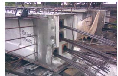
View of Girder after Concrete
