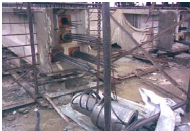
View of Girder after Stressing
