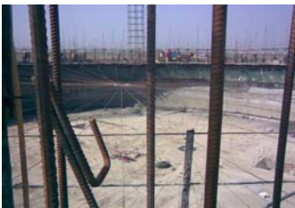
View of Slip Form Spider from Inside
