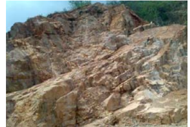
Hill Slopes before Strengthening /Stabilizing
