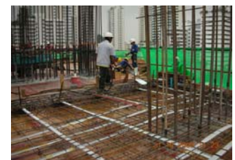
PT Tendon Installation
