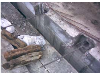
PBL Mono Strand Bonded Tendon System Introduced in Block-A
