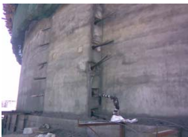
View of Silo During Slip Form
